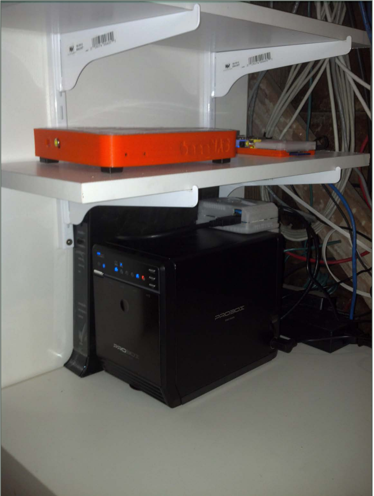
Figure 1. My New Server Rack
